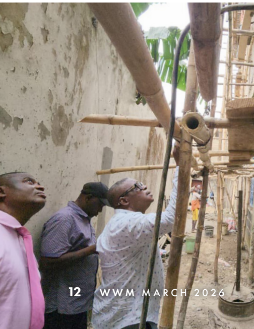
▼ National Administrative Headquarters, Lagos, Nigeria
