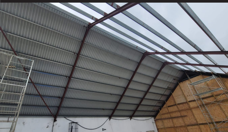
MONTEGO BAY, ST. JAMES - PROGRESS
