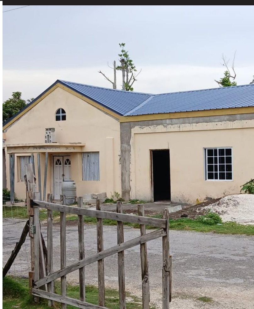
SLIPE, ST. ELIZABETH - PROGRESS
